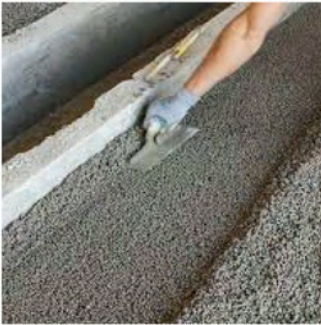
Cement Based Screed Layer
